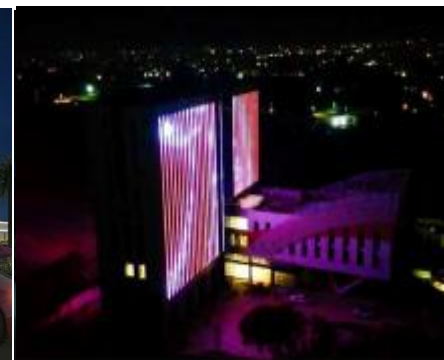
Nile Petroleum New Nilepet HQ, South Sudan
